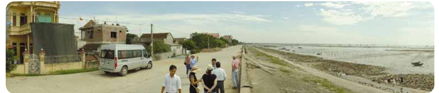
Flood embankment in Hau Loc
